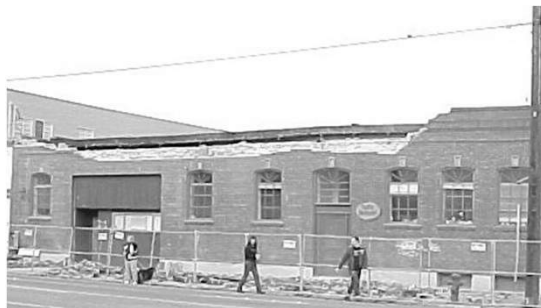
Collapse of an unreinforced masonry parapet
