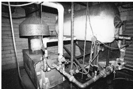
Rupture of water line due to the shifting of a storage tank
