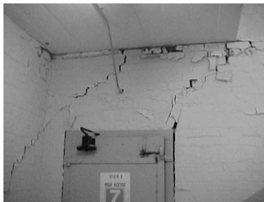
Cracking of heavy masonry partition walls
