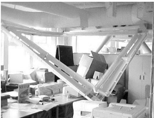
Failures of suspended lighting fixtures in an office building
